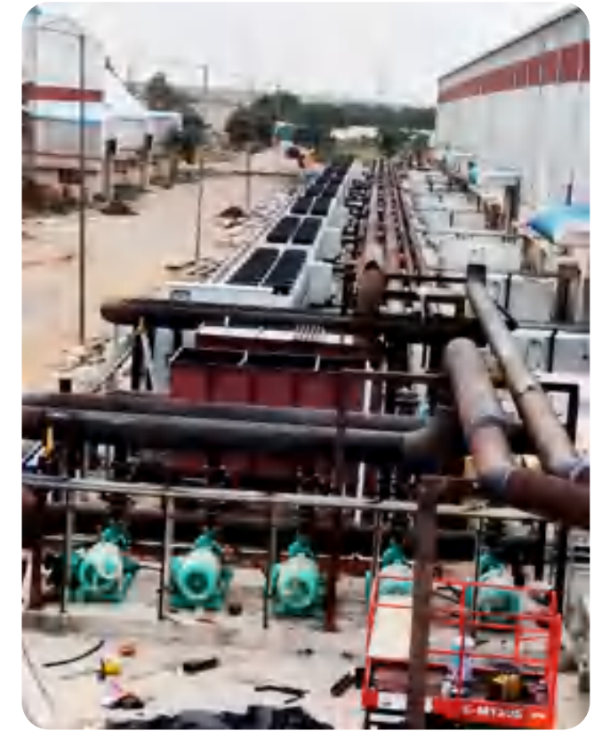
▶ Air Cooled Chiller Plant -3200 TR
