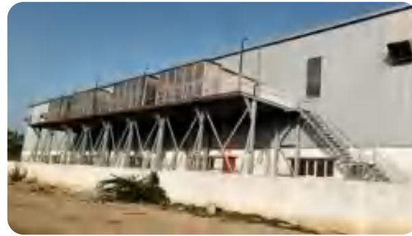
► Two Stage Evaporative (HMX) - 240000 CFM
