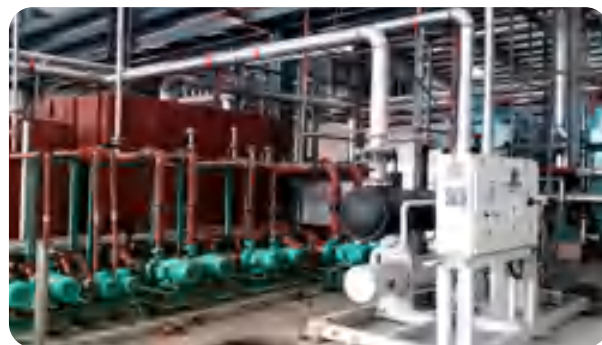
► Process Cooling VAM Chiller-300TR
