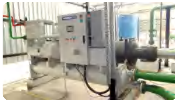
► Water Cooled Chiller Plant (Kirloskar Chiller)- 130 TR
