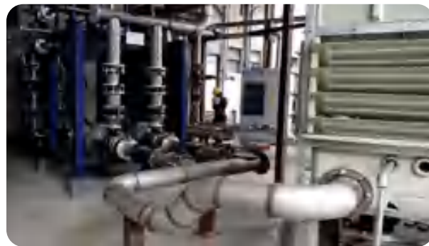
► Water Cooled Chiller Plant (Kirloskar Chiller)-130TR
