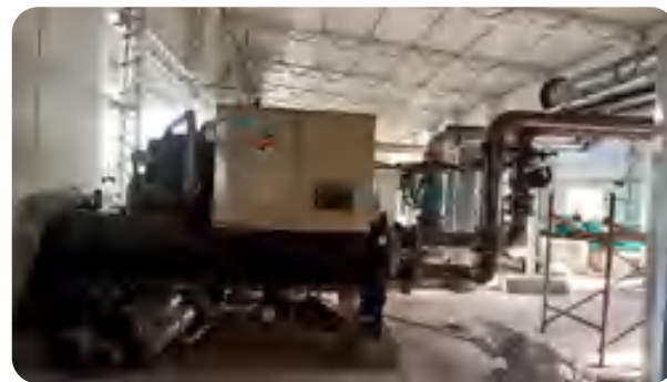
► Chiller Plant - Ice water -300TR (Daikin Screw Chiller)
