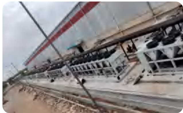
▶ Air Cooled Screw 400TR
