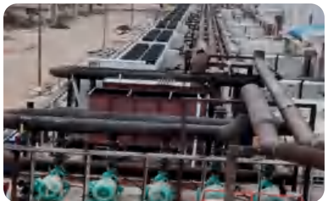
▶ 4200 TR Air Cooled Chiller Plant
