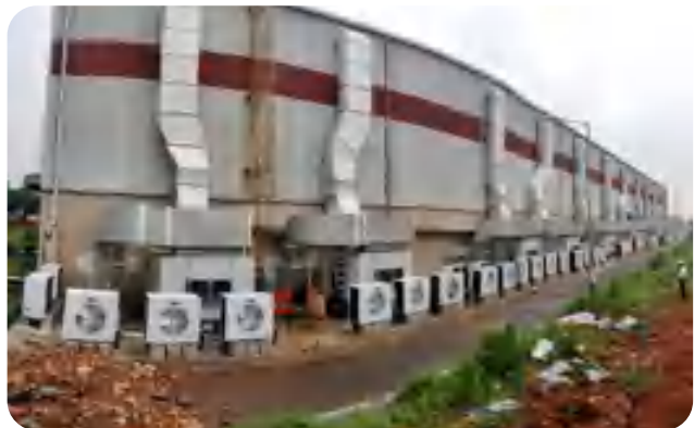
▶ 1000 TR DX AHU System
