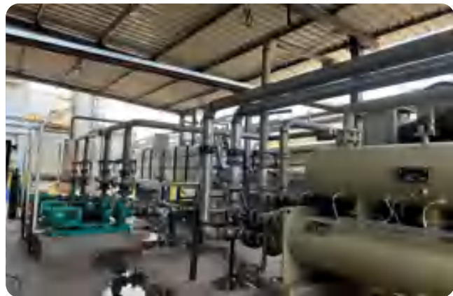
Chiller Plant with SS Pipeline
