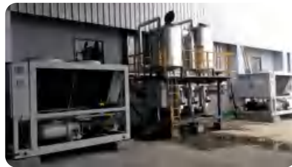
► Process Cooling with Air Cooled Screw Chiller (Kirloskar)
