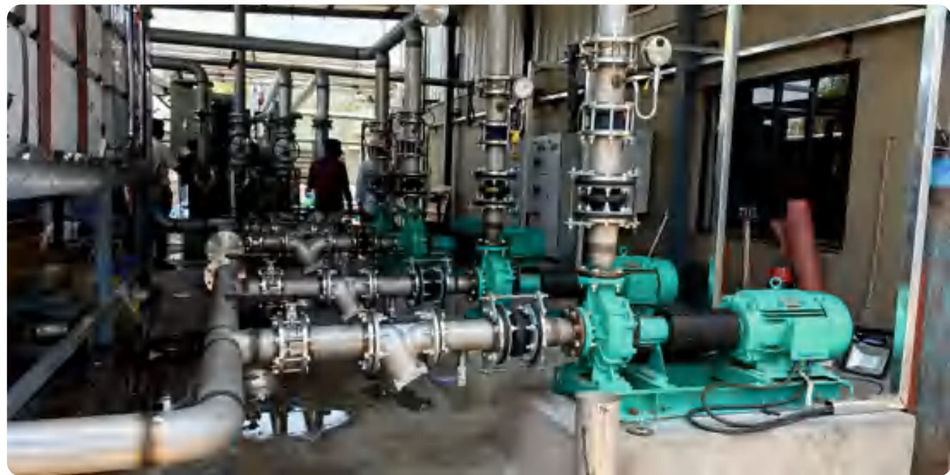
Chiller Plant with SS Pipeline
