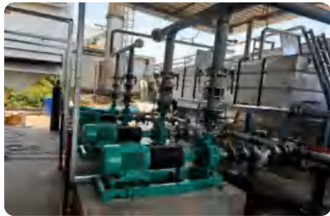
Pumping Station with Hot/Cold well
