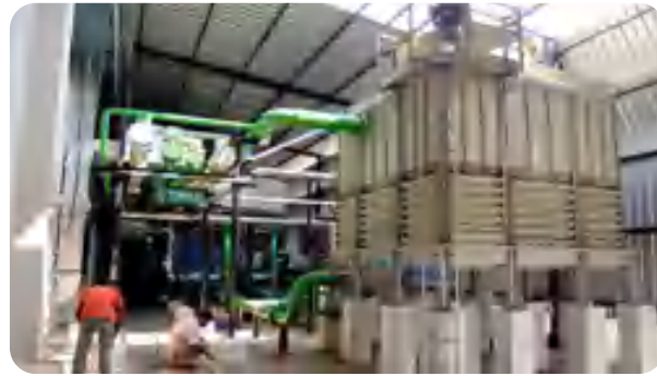
► Screw Chiller Plant -140 TR
