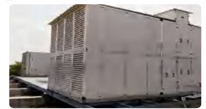
▶ Two Stage Evaporative-30K CFM
