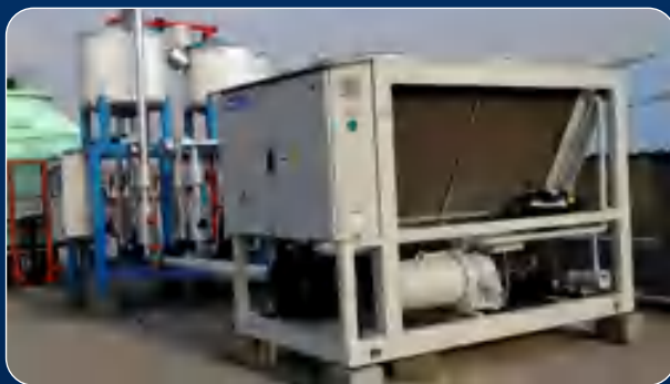
▶ Air Cooled Scroll 50TR Ketchup cooling
