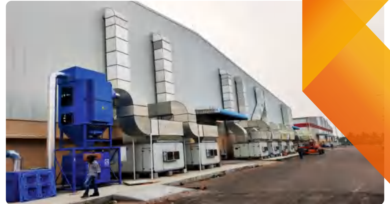
► Chilled water AHU with Lower Return
