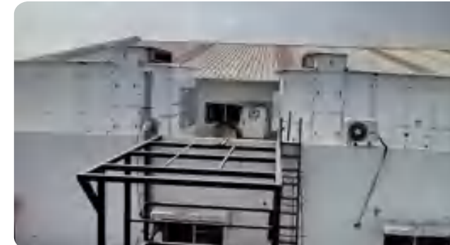
► Two Stage Evaporative- 30K CFM x 2
