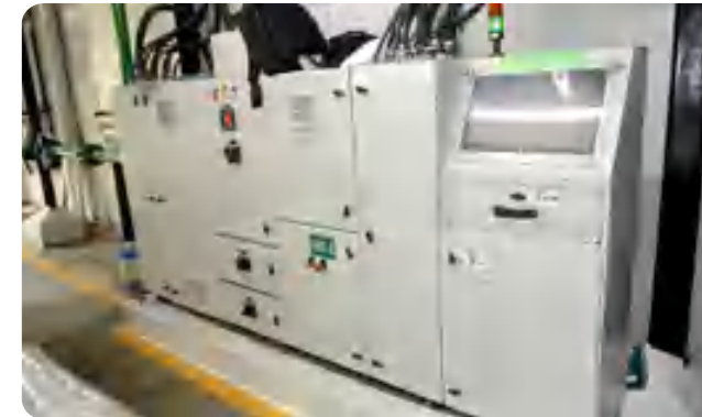
► SCADA Based Electrical Panel
