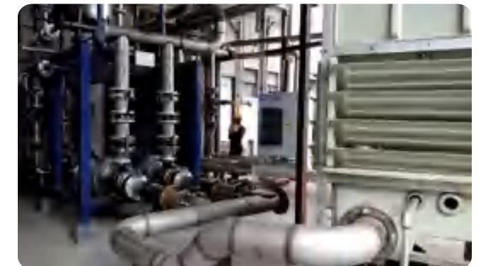
▶ Pump Skid with Hot & Cold well
